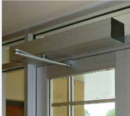
Single—side load lintel mounted header
