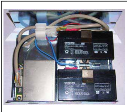
US801105 BATTERY UNIT (2301/2401)
